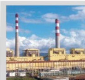
Beilun Power Station in Ningbo
